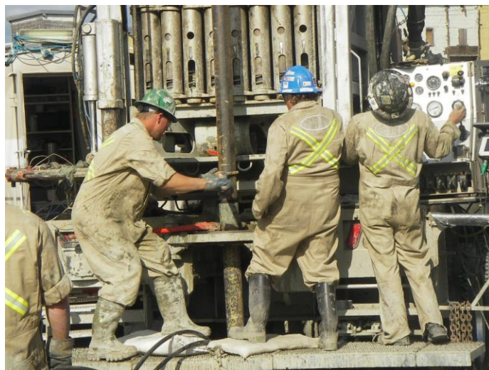
Installing J-55 pipe
