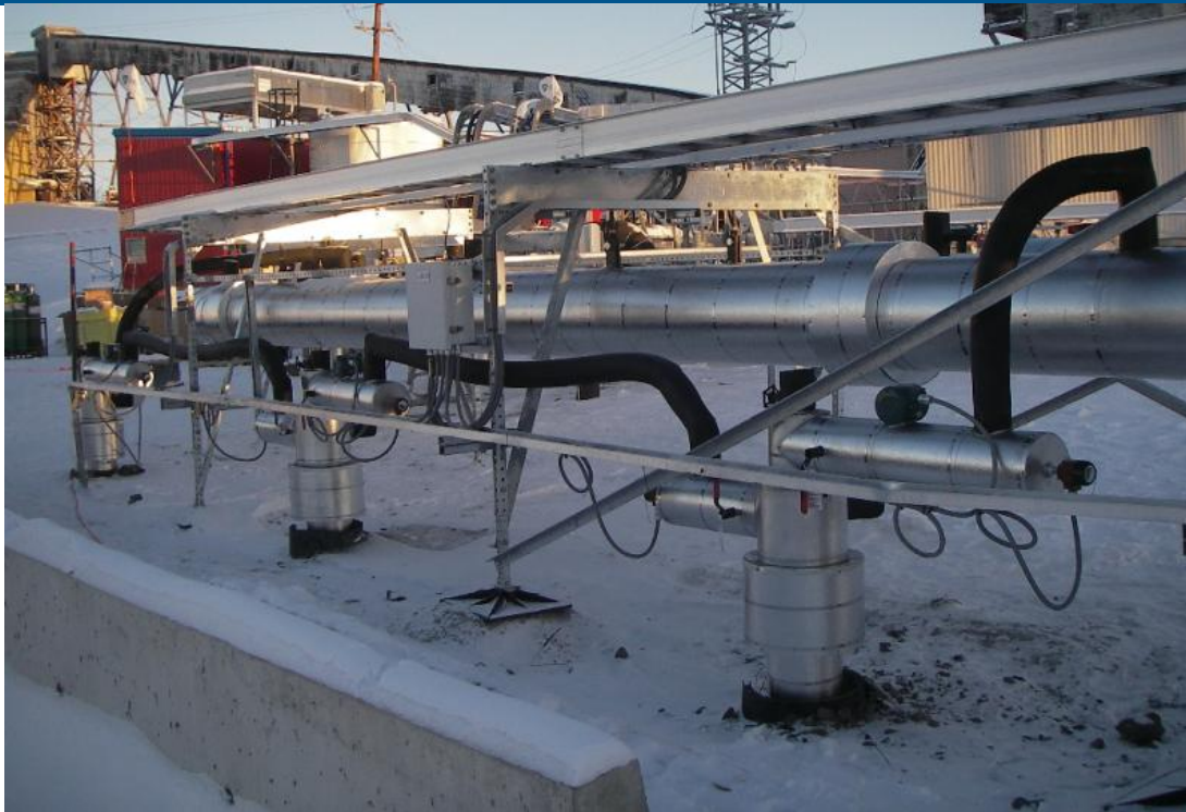
Coolant distribution piping
