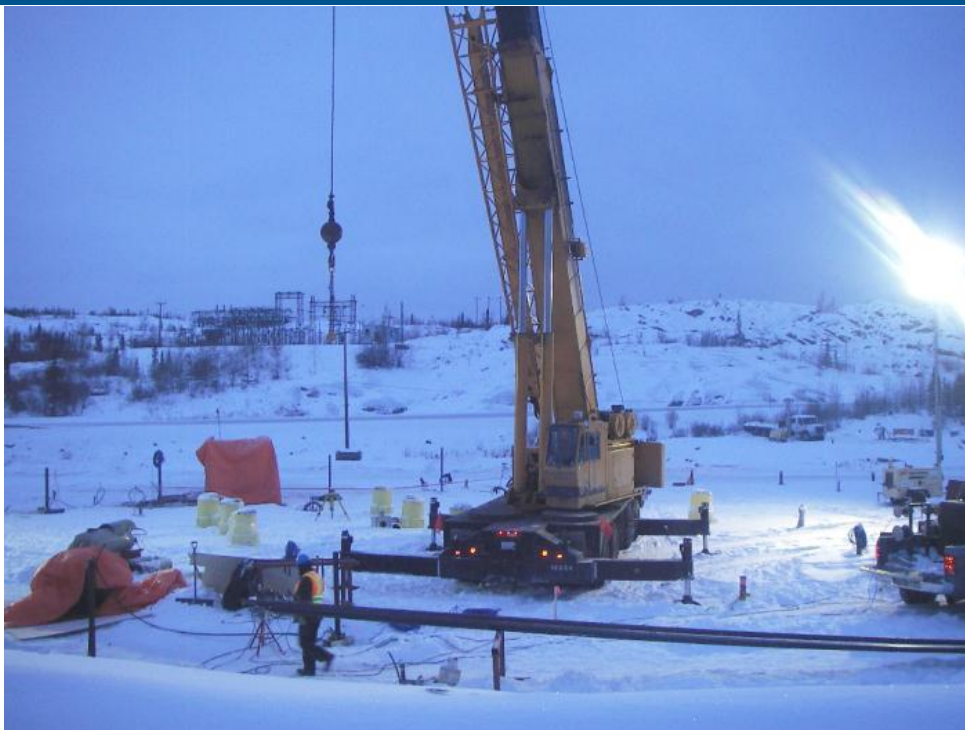
Crane installing thermosyphons
