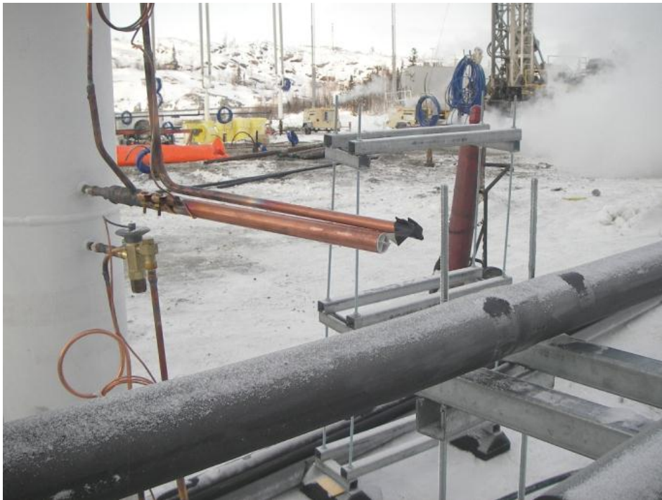
Thermosyphon cooling system
