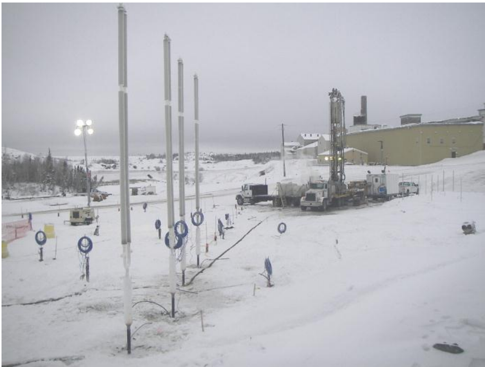
Thermosyphons in place
