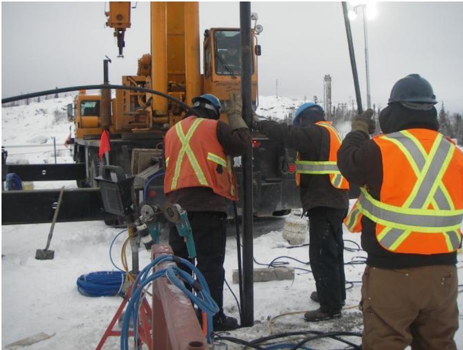
Installing freeze pipe and grout pipe
