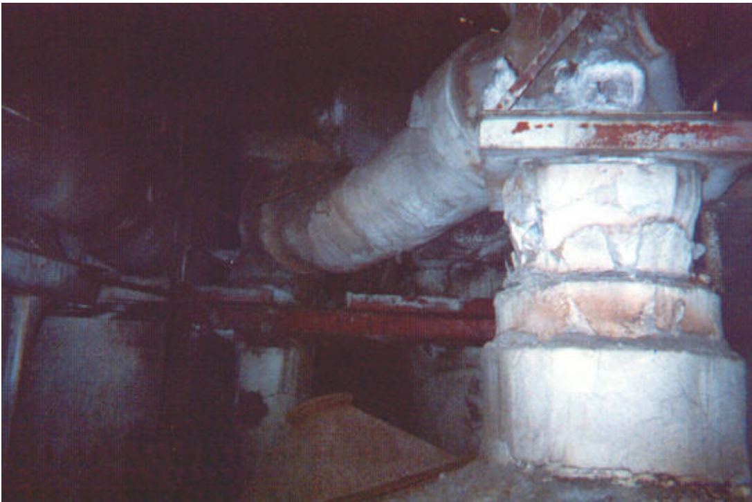
Photo #4: Exhaust flue from #2 roaster vessel to the dust collection cyclones. Note the white crystalline arsenic formation.
