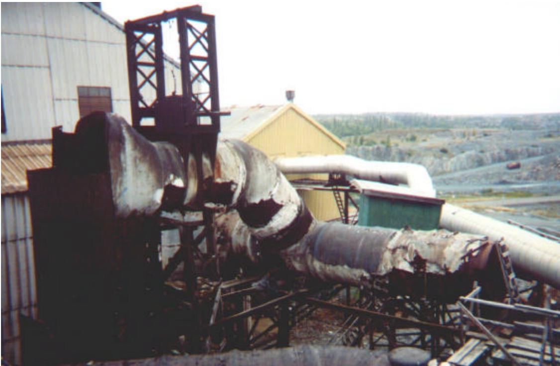
Photo #6: An old flue section that once connected the Cottrells to the stack (pre arsenic baghouse).
