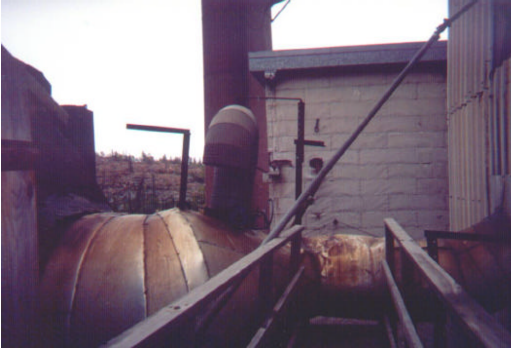
Photo #1: Transition section between roaster and Cottrell. Note change of diameter where the more recent flue replaced a section of much larger diameter old flue.
