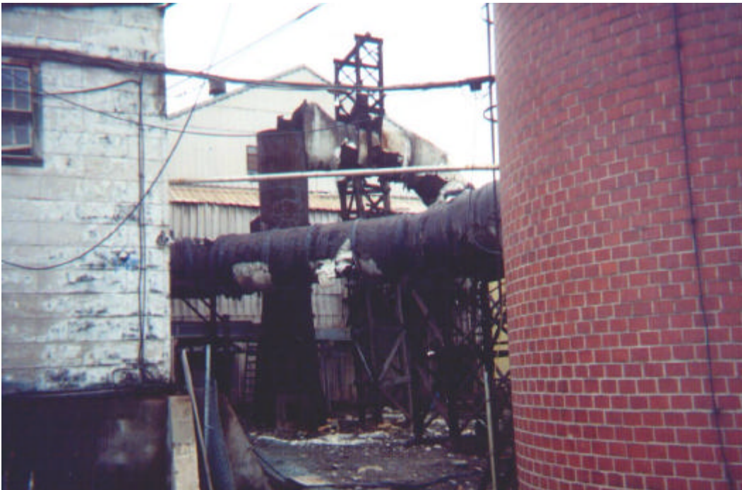
Photo #2: This view shows the base of the brick stack, the 40' high column, and the flue connecting the (no longer existing) AC roaster and the base of the stack.
