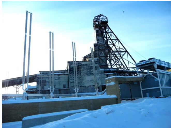
Thermosyphons at Giant Mine
