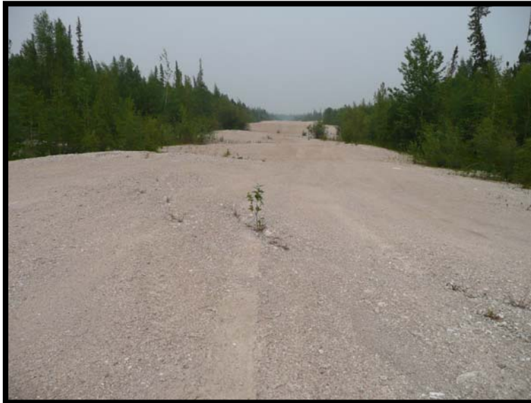
Photo 13 – View of settlement on haul road due to melting of permafrost.
