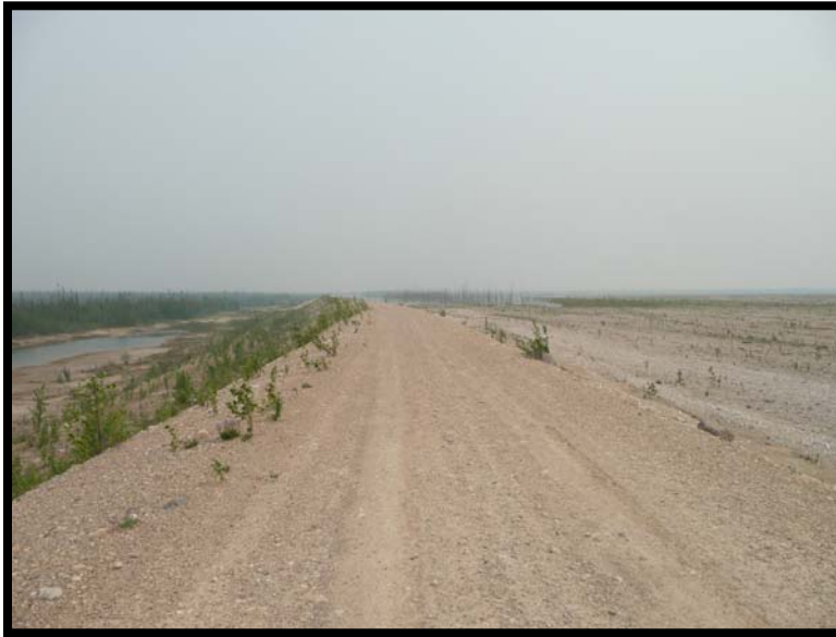
Photo 3 – Cominco tailings embankment and reclaimed tailings beach to right.
