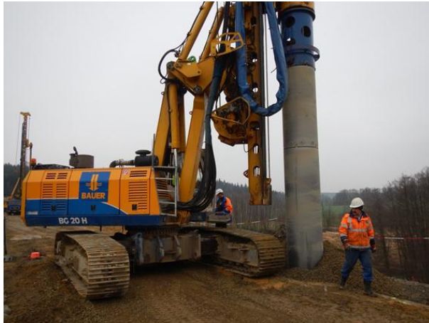
Typical pre-drilling equipment (Rennersdorf, Germany)
