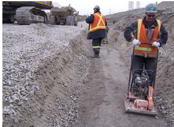
Compaction of Zone 1A material in the toe drain trench.
