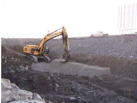
Extension of filter blanket in advance of toe berm construction.
