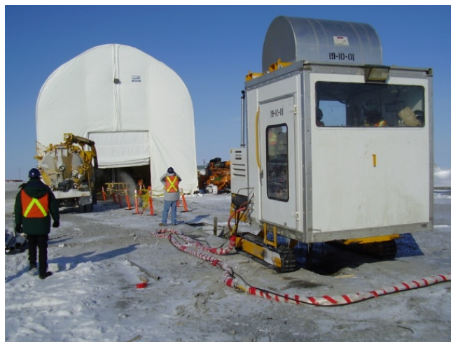
Curtain grouting rig (foreground). Winterized shelter for jet grouting in the background.
