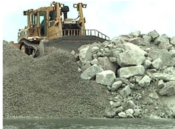
Rockfill being pushed into the lake. To left is Zone 1, to right is Zone 3.
