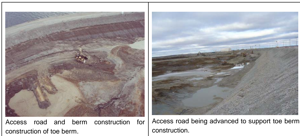
Figure 6-13. Access construction for toe berm following dewatering.
