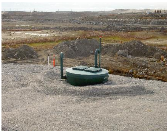
DPS on toe berm of A154 dike.
