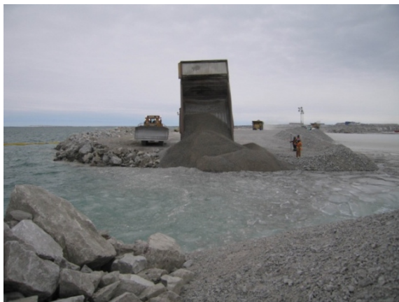
Embankment advancement (nearing closure of the A418 dike). Zone 3 to left, Zone 1 to center (being dumped by truck), Zone 2 to right.
