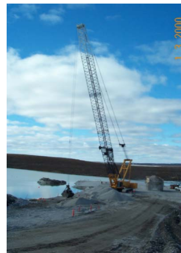
Filter blanket placement via crane and clamshell.
