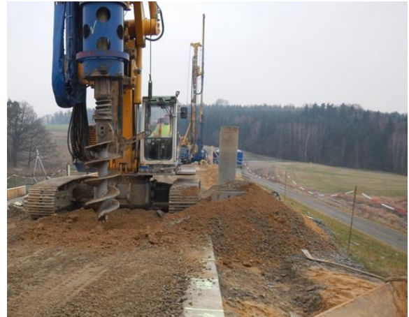
Typical pre-drilling equipment (Rennersdorf, Germany)
