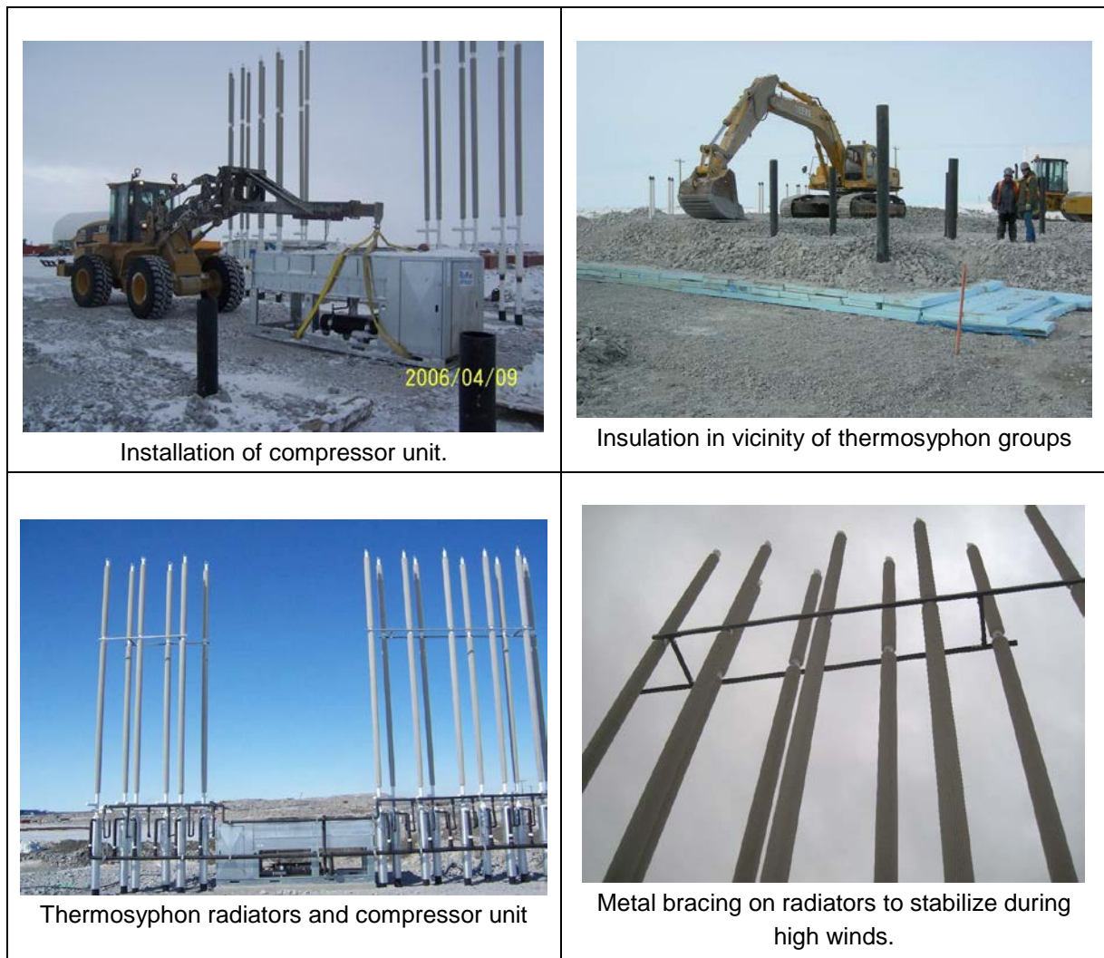
Figure 6-11. Thermosyphon groups.
