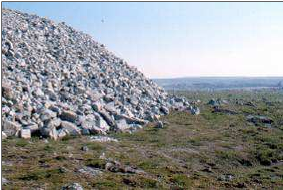
Plate 4.3-1. Typical WRSA embankment (note large fragmentation that encourages cool air flow).
