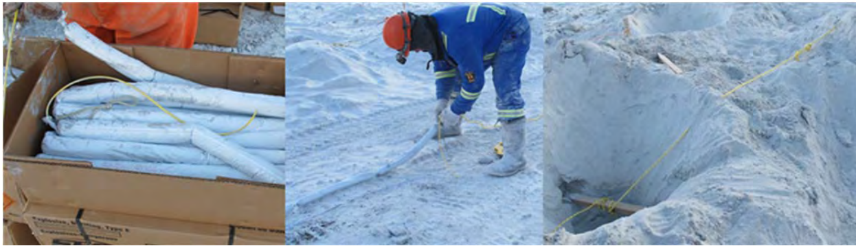
Figure 3-1: Pre-shear Loading
