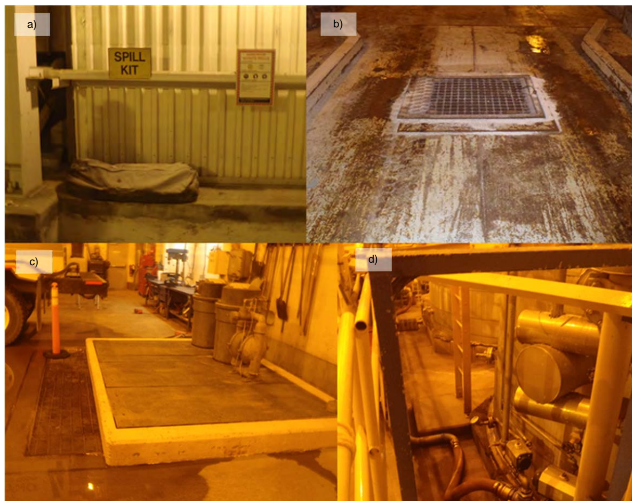
Figure 4-1: Spill Kits and Catchment Basin Examples at the AN Storage Facility and Emulsion Plant
