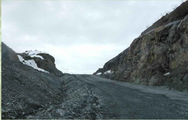
EXAMPLE OF A ROCK "THROUGH CUT" WHICH IS PROPOSED ON THE APPROACHES AT KP 23.5 AND KP 25.4 CROSSINGS
