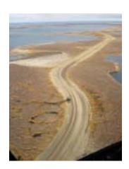
Permafrost underlies about half of the landmass of Canada and our northern road, rail and air transportation system is reliant on the strength of permafrost soils. Defined as a ground condition of either soil or rock that remains at or below 0°C for long periods, permafrost is often a very capable foundation but it is very sensitive to changes in thermal conditions.
