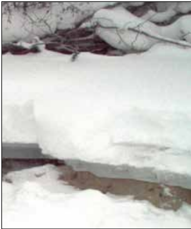
Figure 4.7: Cracking along the shoreline of a lake following significant drop in water level.
