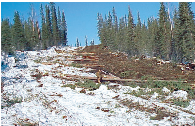
figure 20. Brush can be used as a sediment trap on steep slopes.
