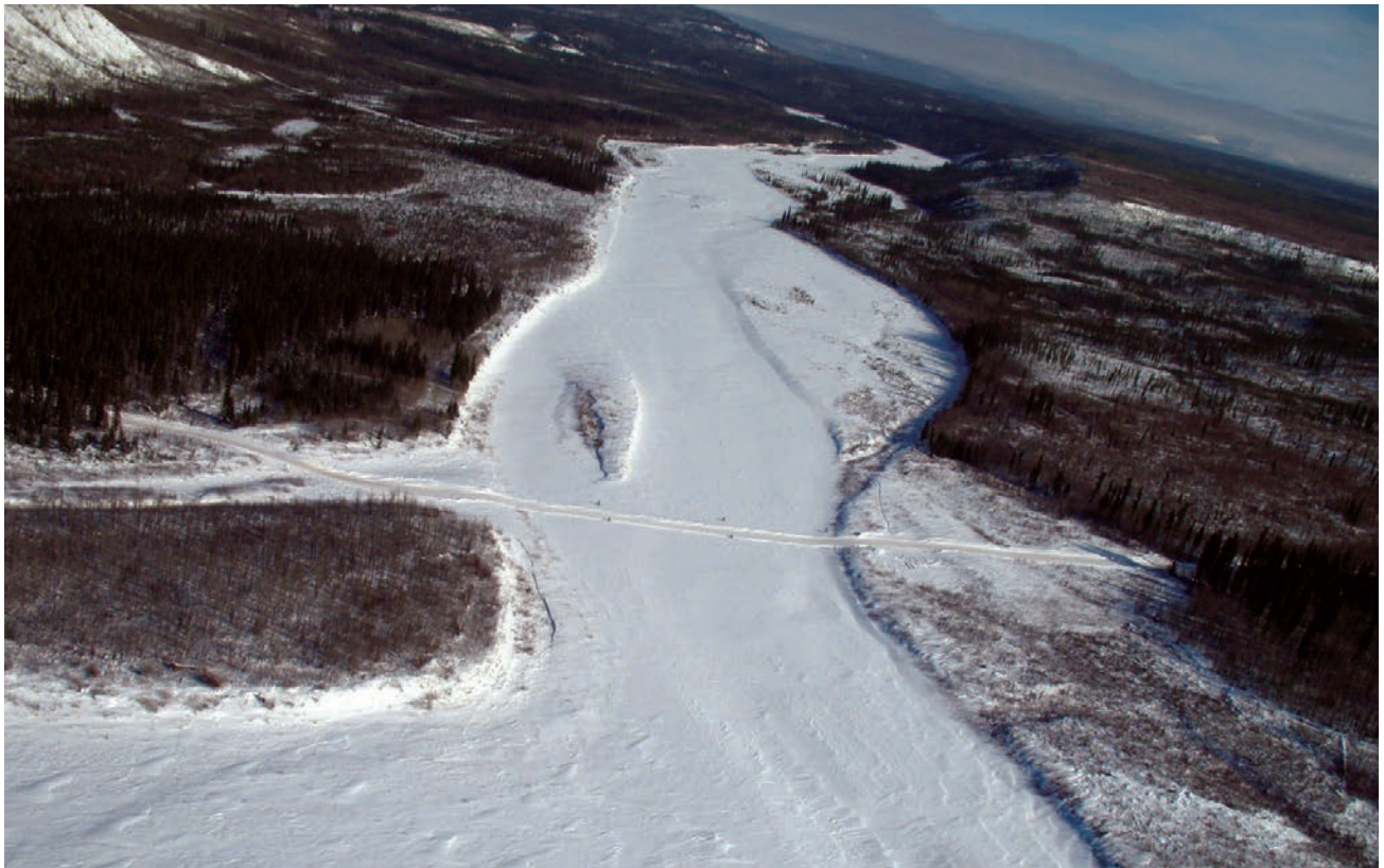
figure 41. An ice bridge built over a large stream channel.
