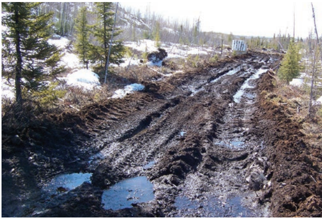
figure 15. Proper scheduling of road construction will avoid rutting and erosion.
