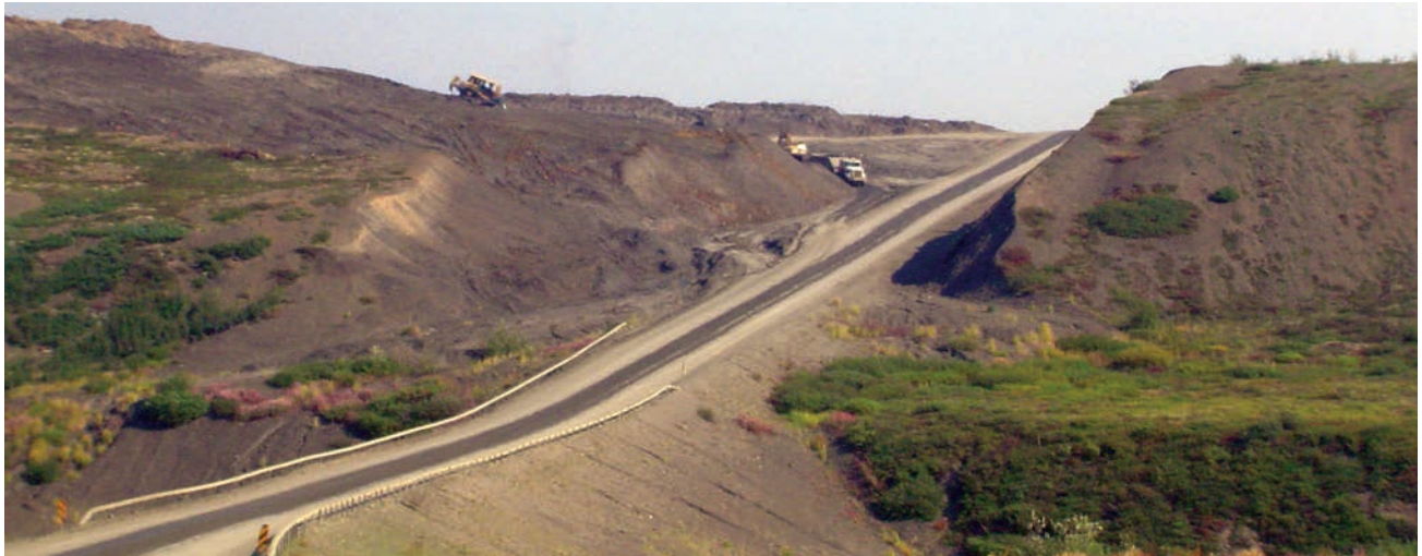
figure 22. The slope of this road has been reduced by fill excavated from the adjacent cut.
