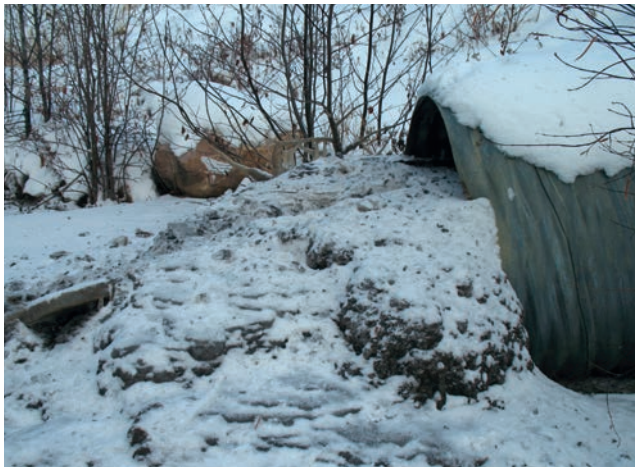
figure 44. Culverts should be monitored and cleaned regularly to ensure that they continue to function properly.
