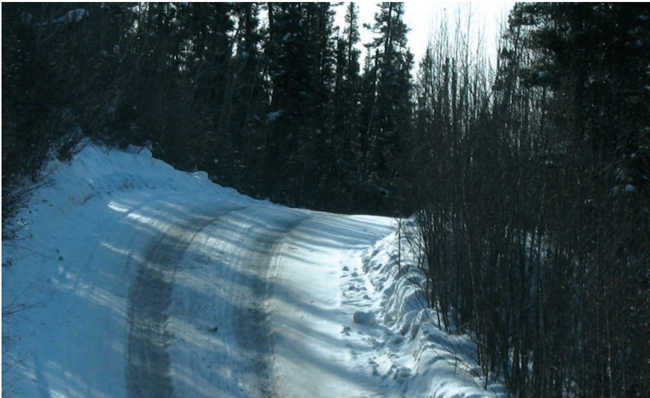
figure 12. Road grades and curves should be designed to be safe and minimize environmental disturbance. In this case, a wider curve and a lower grade would be safer and less prone to erosion.
