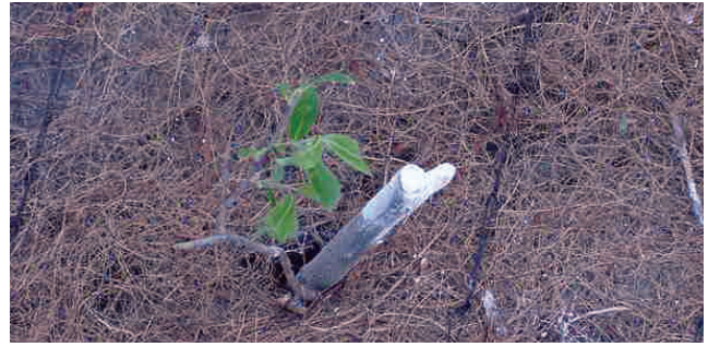
figure 51. Erosion control can include the use of mats and planting willow cuttings.
