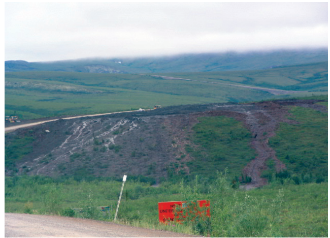
figure 45. Regular monitoring will identify areas where drainage controls are inadequate and need to be redesigned.
