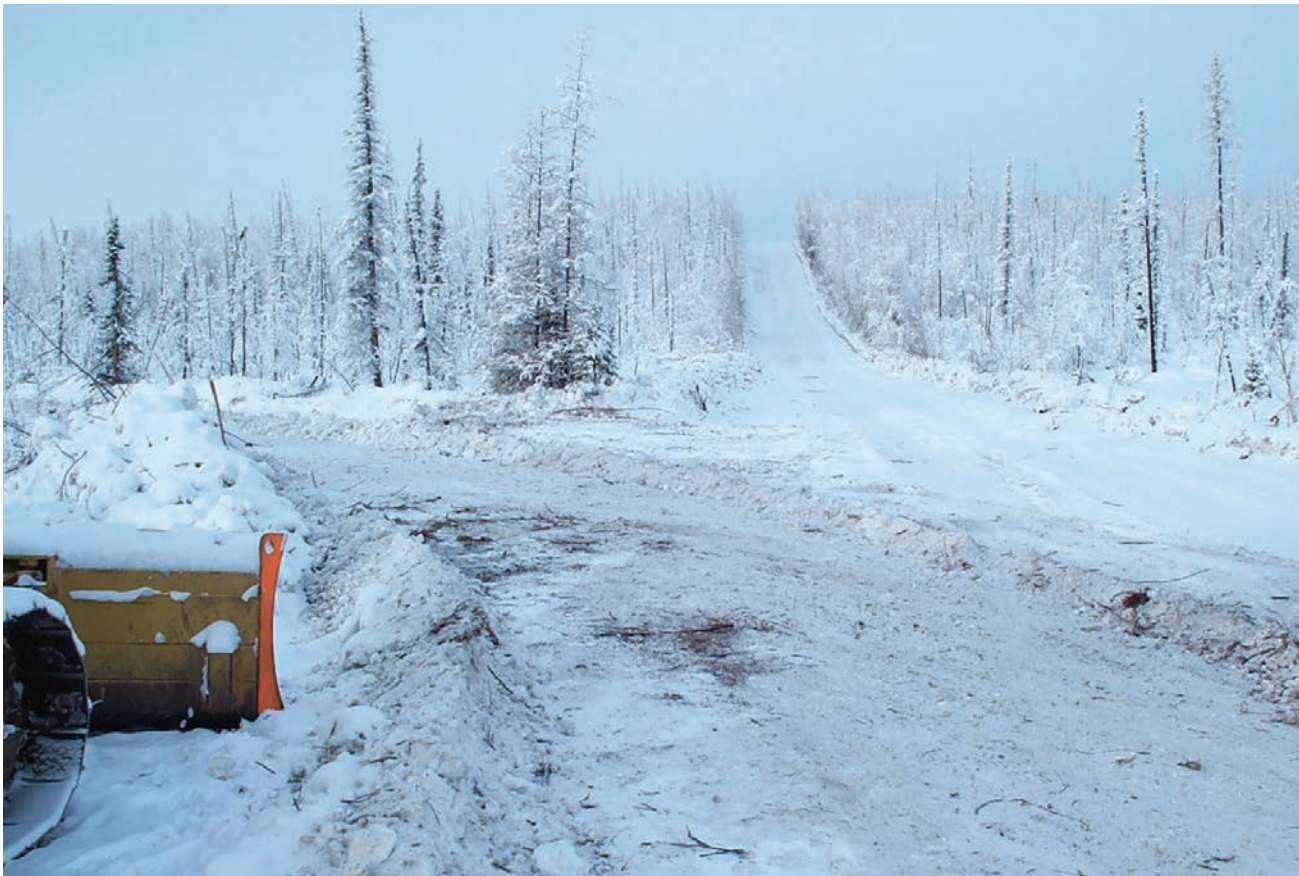
figure 14. Verifying the route prior to construction can avoid unnecessary false starts such as this one
