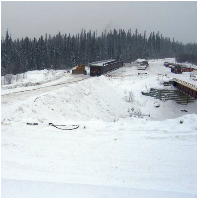
figure 39. A well-constructed snow fill located adjacent to a new bridge.
