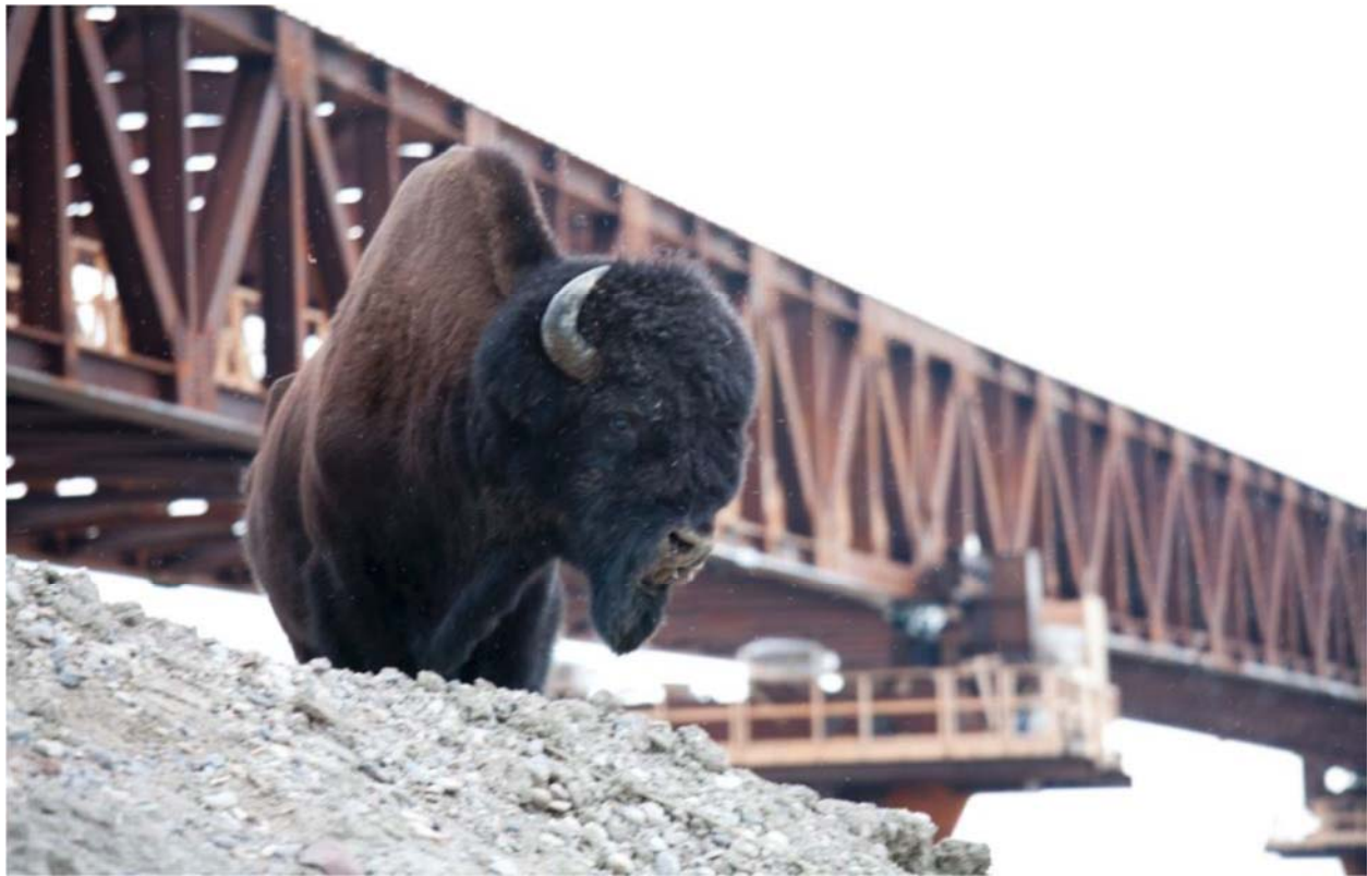
Figure 10-4. Bison at Deh Cho bridge during construction, 2011.
