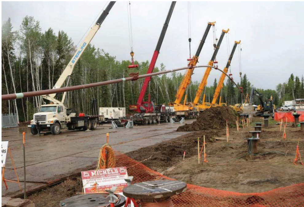
Figure 10: Enbridge pipeline replacement at Mackenzie River crossing, 2018 GNWT inspection report photo
