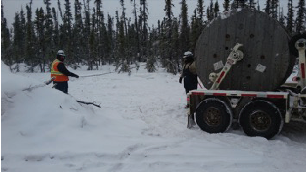
Figure 6: Trenching and laying the Fibre optic cable along the Mackenzie Valley, March 2016
