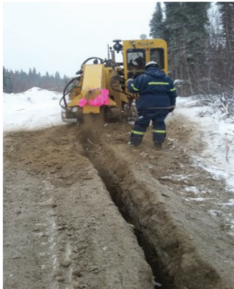
Figure 6: Trenching and laying the Fibre optic cable along the Mackenzie Valley, March 2016
