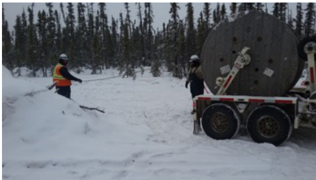
Figure 6: Trenching and laying the Fibre optic cable along the Mackenzie Valley, March 2016. Review Board photo.
