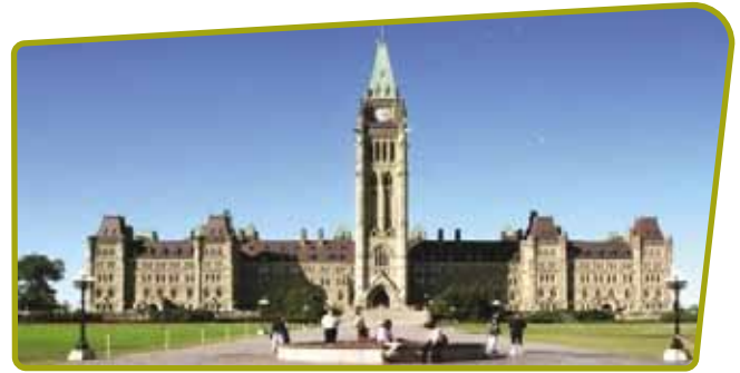
Parliament Buildings, Ottawa. This is where the Gwich'in, Sahtu and Tlicho land-claim agreements, and the MVRMA became law. Photo copyright Parks Canada
