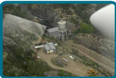
An ariel shot of the Taltson Twin Gorges hydroelectric plant.
