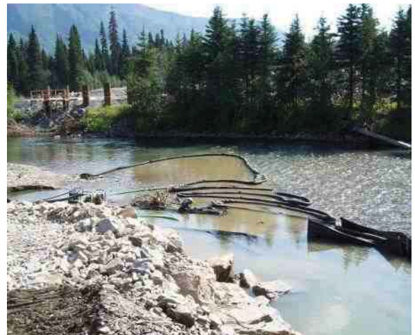
Figure C-5. Instream sediment curtain application for rip-rap installation in a low gradient shallow stream channel
