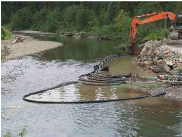
Figure C-5. Instream sediment curtain application for rip-rap installation in a low gradient shallow stream channel
