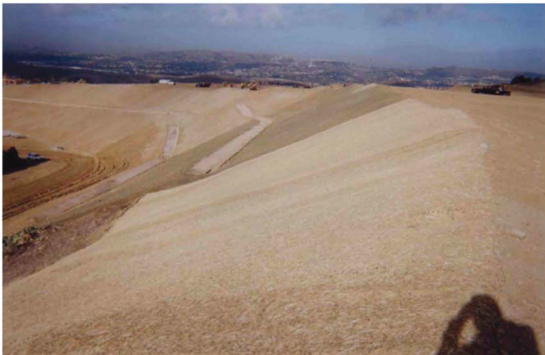
Figure EC BMP #4.2. Rolled Erosion Control Products: Slope Installation
