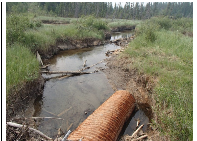
Photo 16: Crossing 8 looking west (upstream); grassed floodplain and organic substrate; note eroded banks with some undercutting (July 3, 2014)
