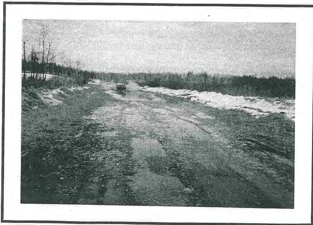
Ponded Water As Daily Mean Temperatures Approach 0°C is a Sign Road Closure is Near
