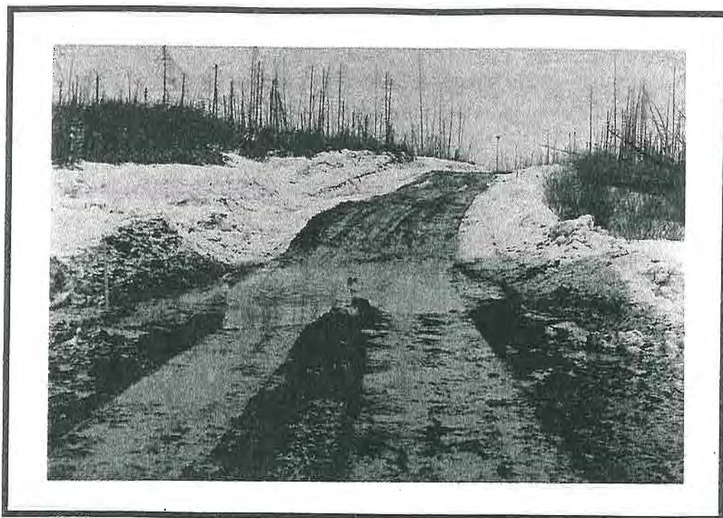
Allow Sufficient Time In Spring For Road Closure Without It Resulting In Unnecessary Terrain Damage.
