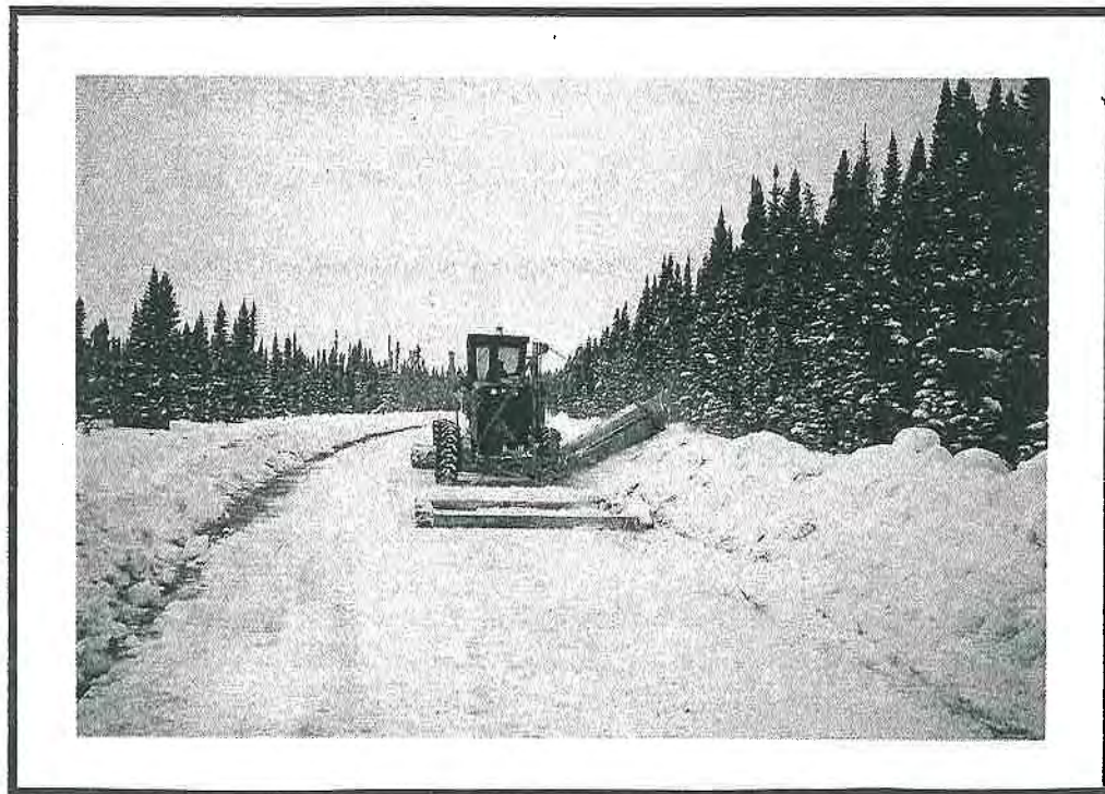
There Is A Fine Line In Compacting Snow That Will Strengthen Under Traffic As Compared To Being Destroyed.
