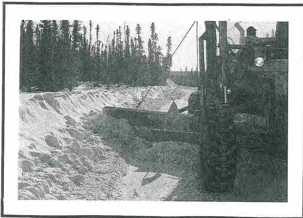
Too Much Snow Can Be Winged Off The Winter Road By Grader To Be Brought Back On Later And Compacted.
