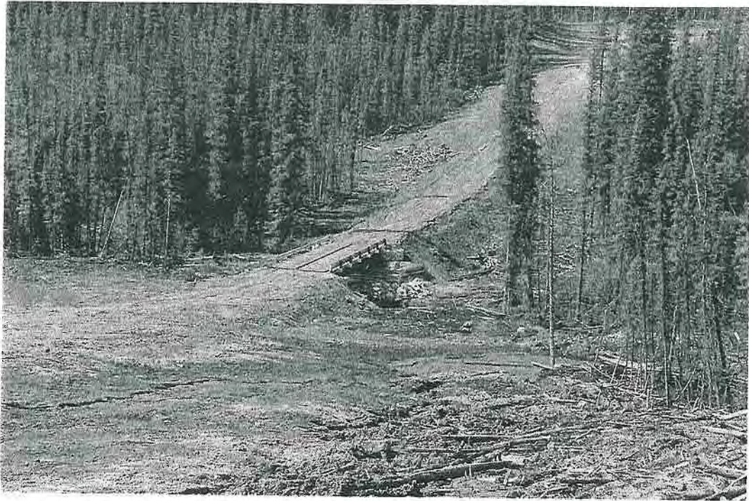
Permanent Bridges On Winter Roads Should Be Properly Designed & Planned as Shown To Possibly Become Part Of A Permanent Road System.
