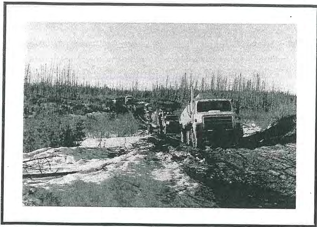
This Winter Road Should Have Been Closed Earlier As There Is No Compacted Snow or Ice Protecting the Terrain, and Rutting is Occurring.
