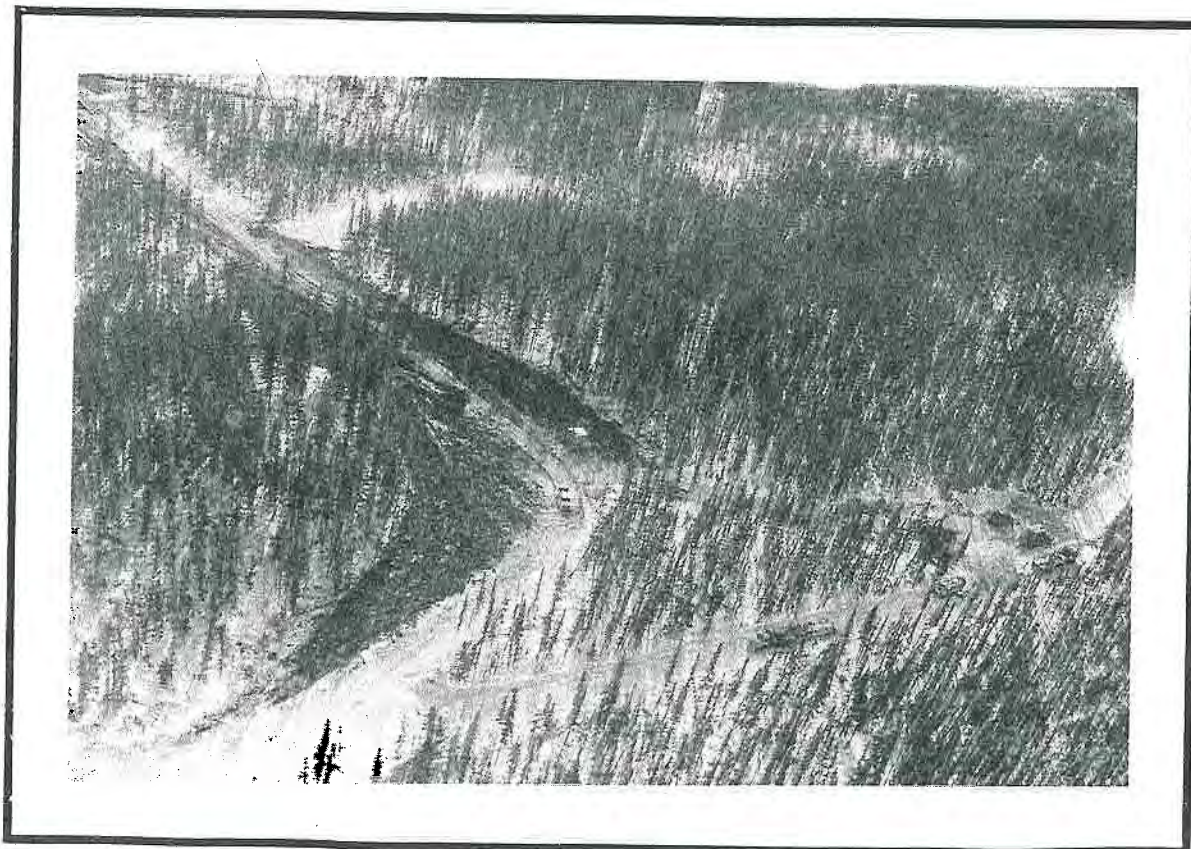
Widening the Right-of-Way at Corners Improves Safety By Reducing Degree of Curve and Improving Sight Distance.
