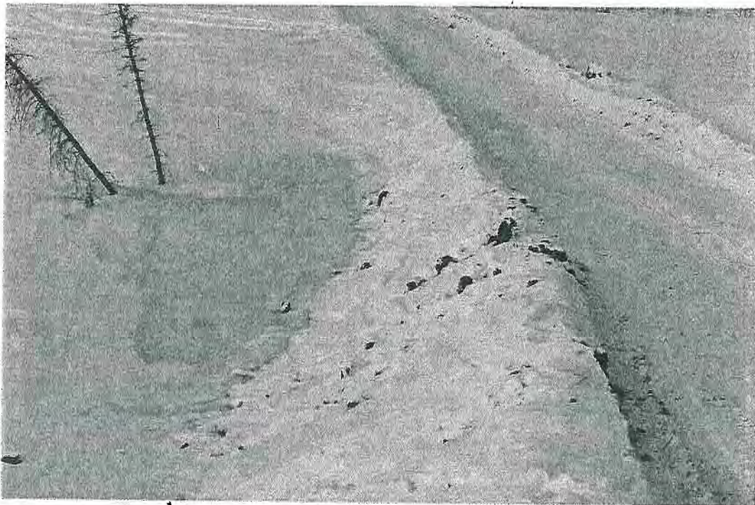
Snowfills Alone (Without Culverts or Corduroy) Should Only Be Used Over Dry Stream Beds And Removed In Spring, to Avoid Interfering With Fish Passage
