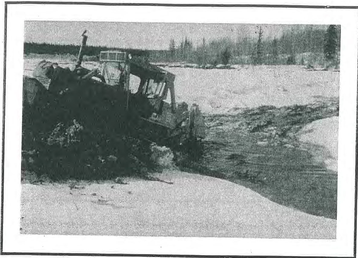
Backhoes Rather Than Dozers Should Be Used To Remove Snowfills. Disturbing Banks Or Bottom Should Be Avoided.
