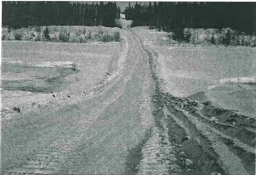
Ice Bridges Provide River Crossings by Providing Naturally or Artificially Thickened or Strengthened Ice Surfaces
