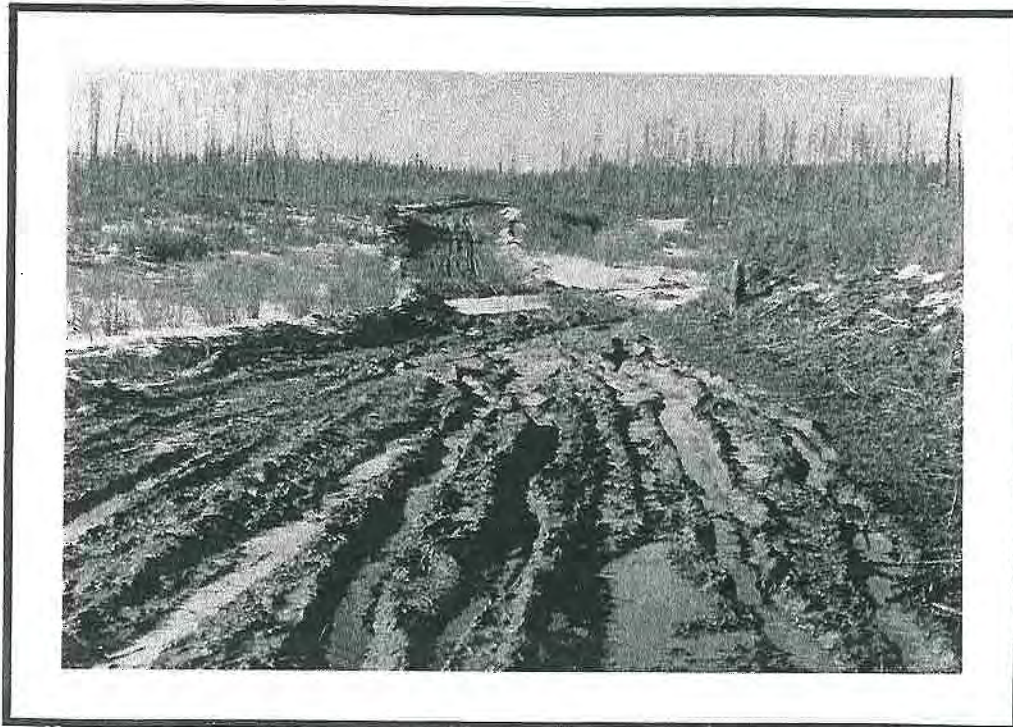
Or, Using Them Too Late In the Spring Is Generally the Cause of Most Environmental Damage.
