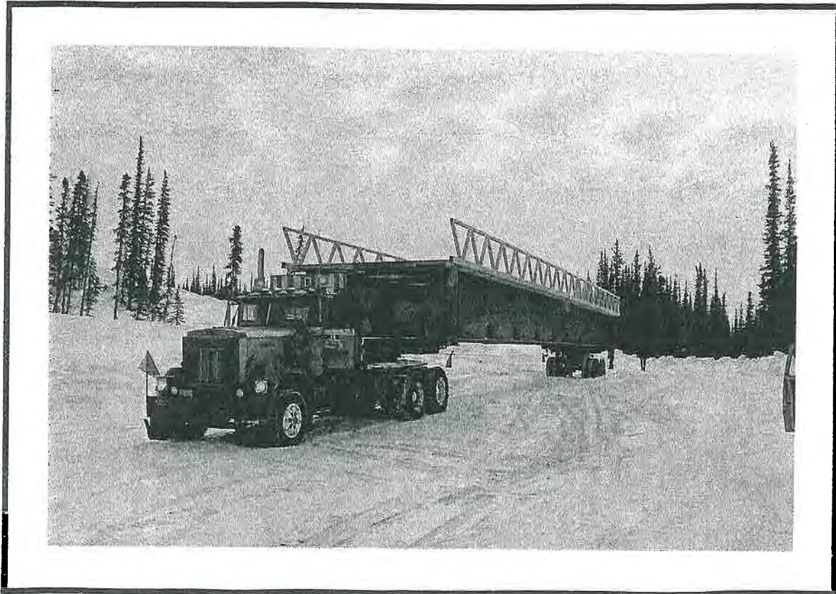
Use Of Structural Single-Lane Bridges Is Unique To DOT's Winter Roads In the Northwest Territories.
