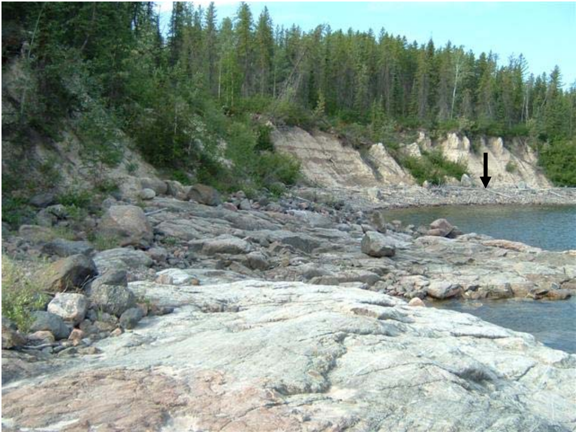
Photo 2.3 Cobble and boulder toe armouring (July 9, 2008).
