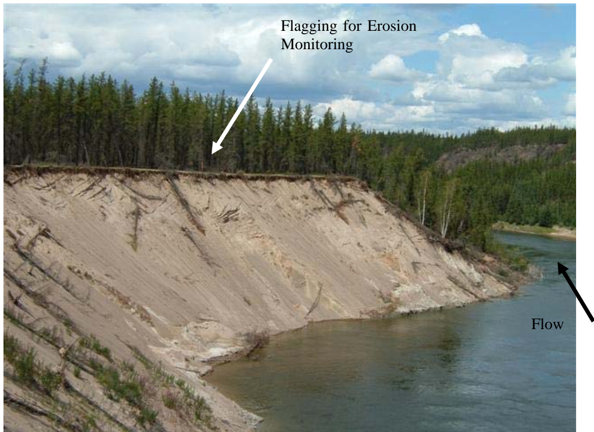
Photo 2.4 Looking downstream at Site 1 where there is no toe armouring (July 9, 2008).
