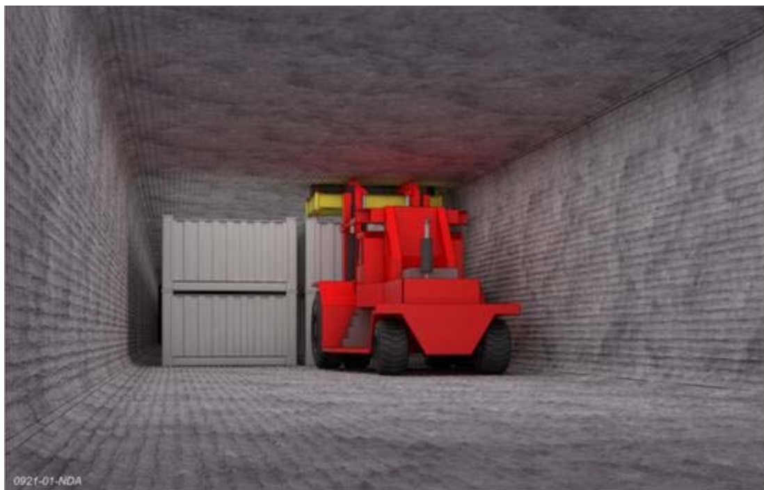
Figure 5.2 Emplacement of shielded ILW packages in evaporite
