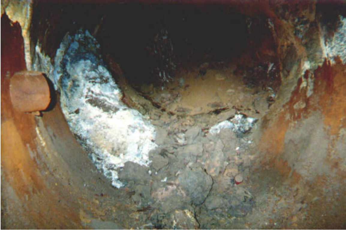
Photo # 7: Flue section in roaster building. Note nipple for air lancing blockages.
