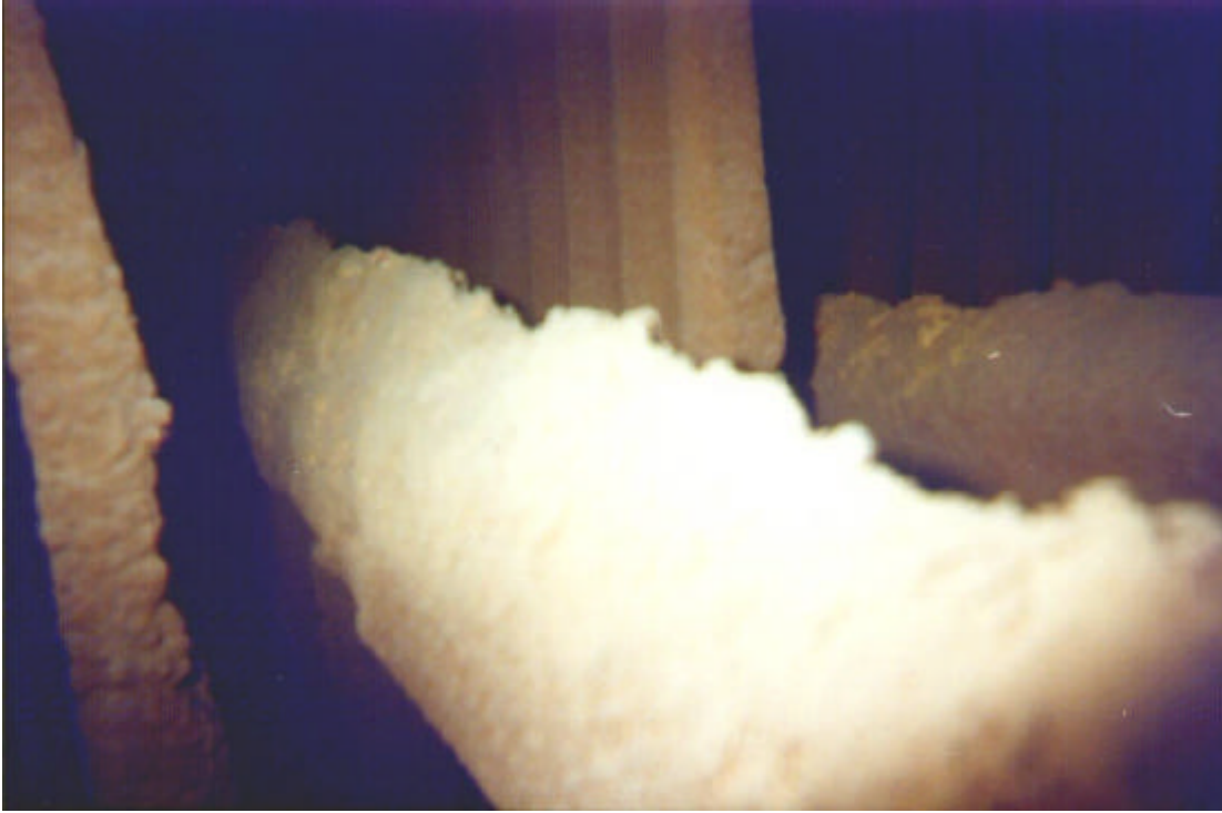
Photo #9: Inside #4 compartment of Cottrell. Note heavy dust buildup on frames between Rod curtains
