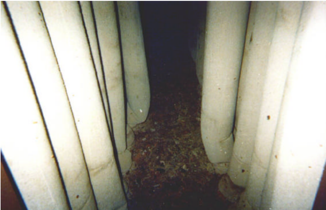
Photo #10: #6 baghouse compartment. Bags are in good condition and the compartment relatively clean. Dust collects on the inside of the bag in this type of collector.
