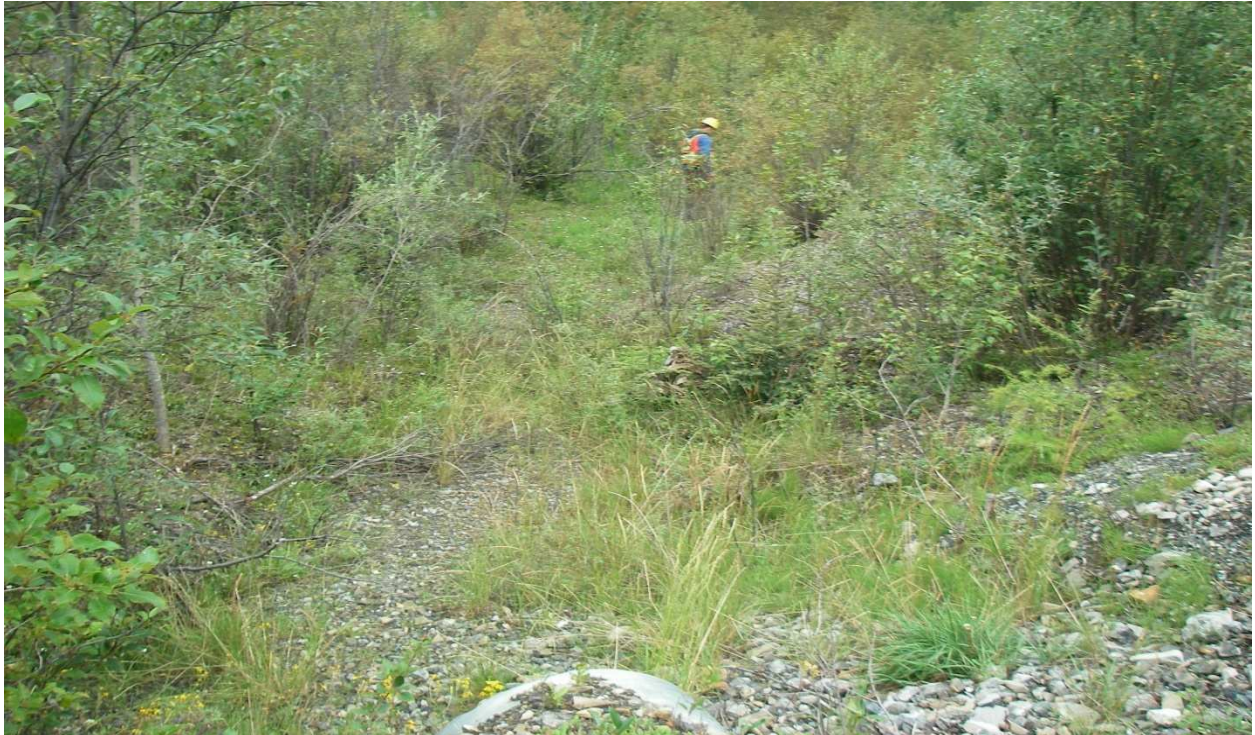
Photo 2. Upper pond basin showing lack of water flow/depth. Note outlet of culvert at bottom of photo.
