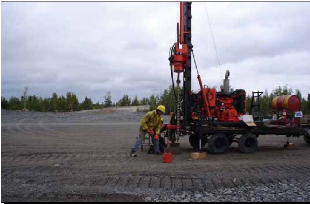
Photo 2 Removing armour rock at BH-17, north end of airstrip
