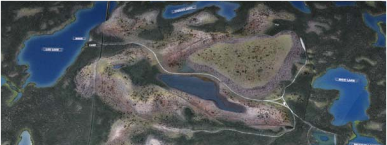
Photograph 3-3 shows the proposed mine closure like looking straight down from an airplane.
