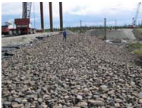
Photo 4: Air Convection Embankment (ACE) – Fairbanks Alaska
