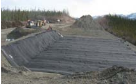
Photo 5: Heat Drain – Beaver Creek, Yukon
