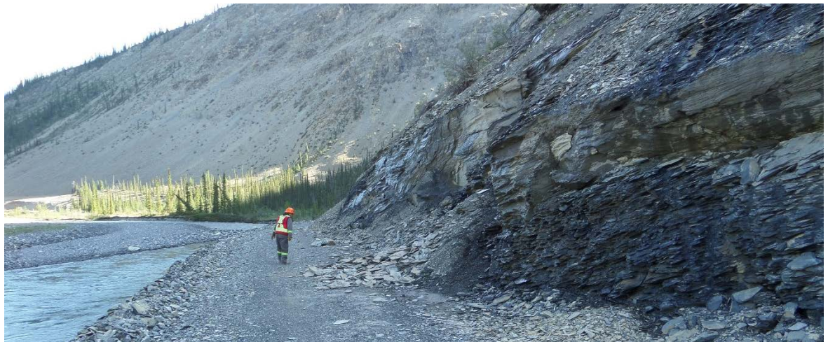
Figure 5: The rockfall hazard at 4.01 km may generate a large quantity of waste rock that could be used to supply subgrade borrow needs elsewhere nearby.
