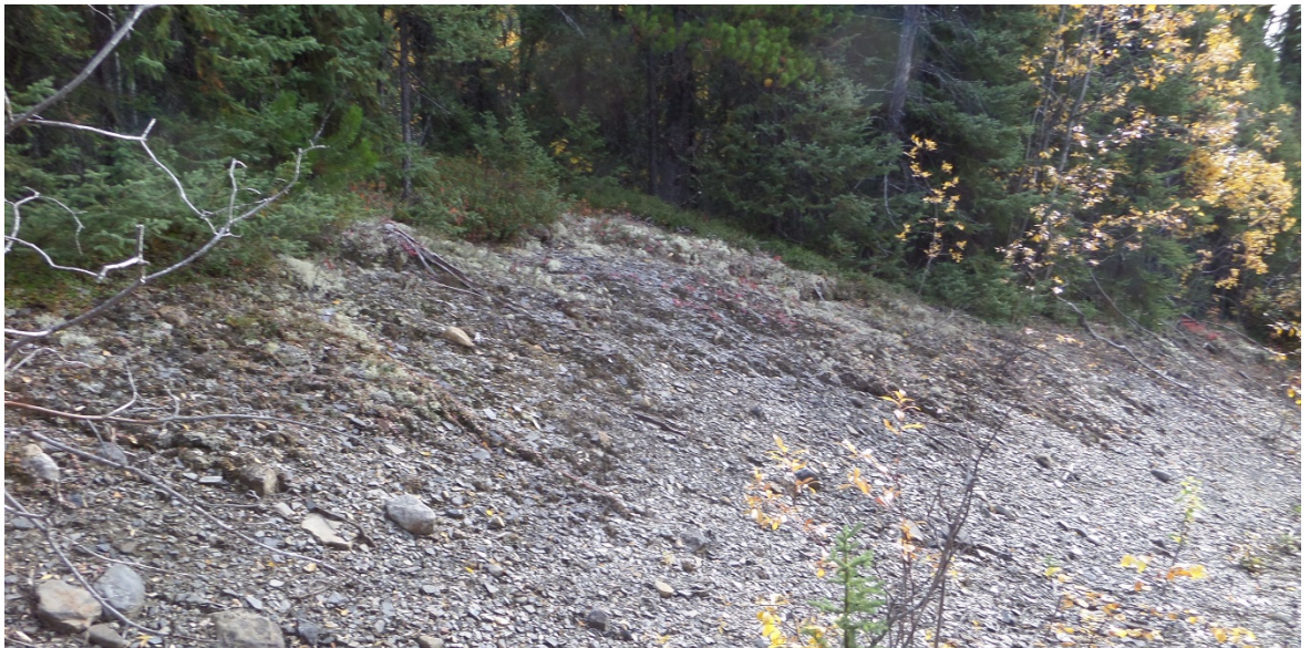
Figure 46: The existing cut slope at BP70. The weathered face appears to be colluvium shale because of the residual fragments left in place, but the slope is in sandy materials.
