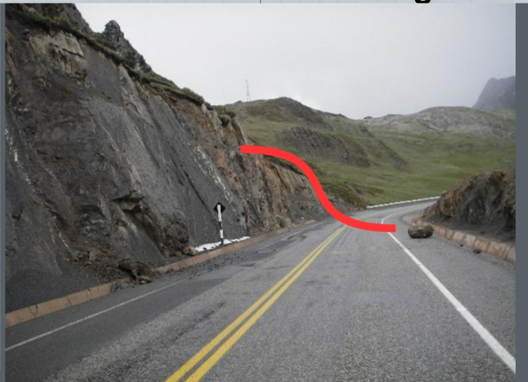
Hazardous rockfalls can occur on well designed and carefully built man-made slopes, like those of Road #2
