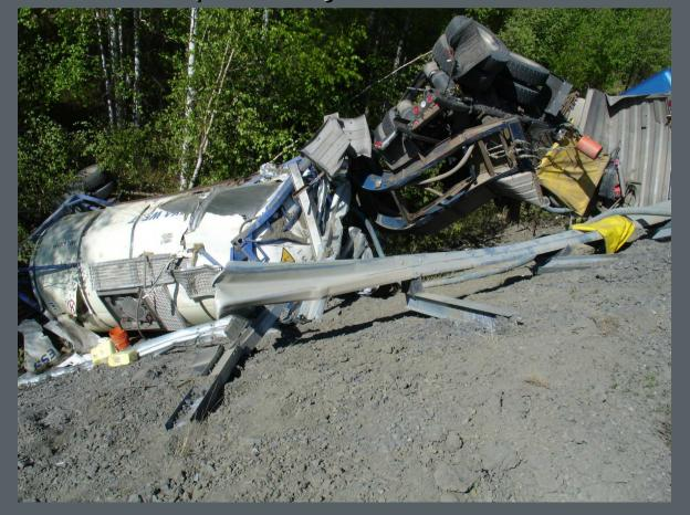
See what happened to this barrier which was neither sufficient nor correctly founded/ anchored in the road shoulder.
