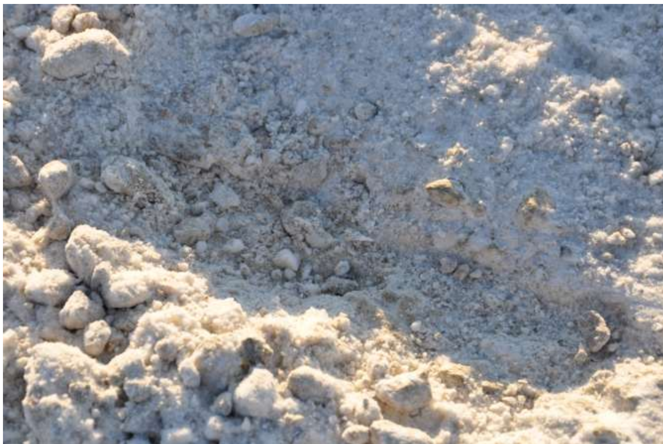
Figure 22: Victor Mine Roadbed Showing Frozen, Consolidated Aggregate in Wintertime [total depth ~4cm] (photo: A Pickup)
