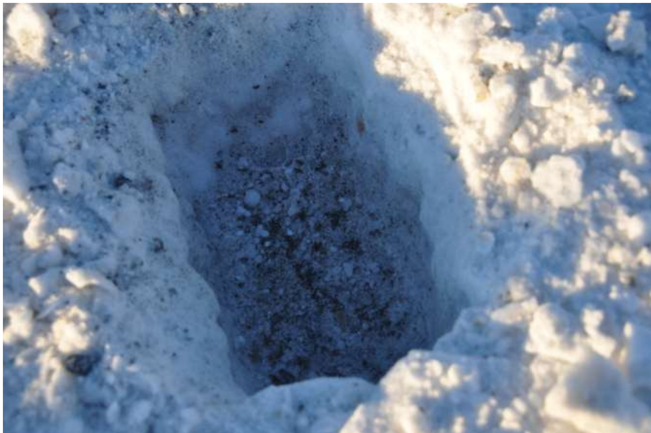
Figure 23: Snap Lake Road Bed Profile Showing Frozen Aggregate and Solid Ice Layer Below (A. Pickup)
