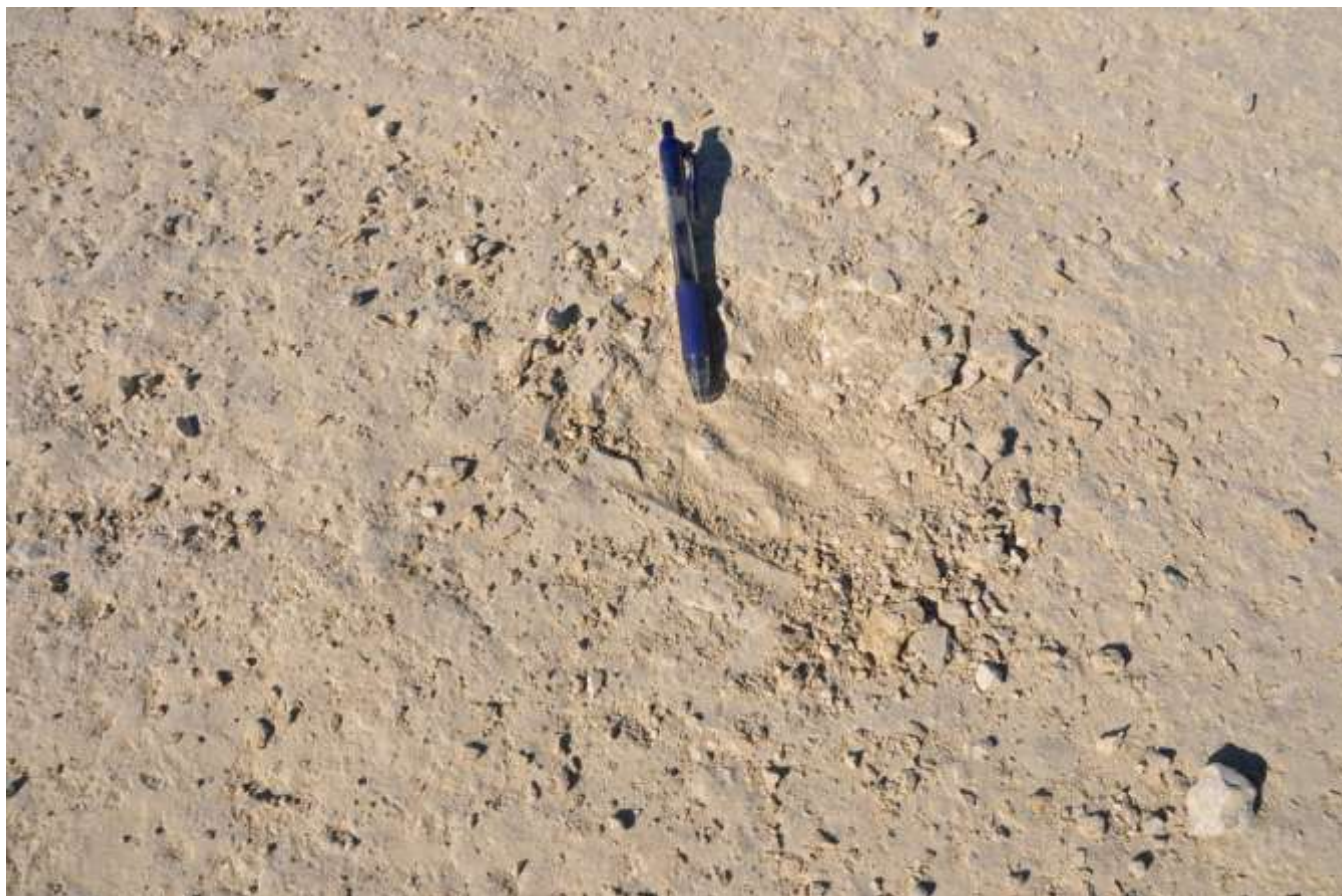
Figure 21: Victor Haul Road Showing Durable Lime Mud Hard Pan, Pen Denotes Area Excavated With a Steel Pick Axe (Photo: A Pickup)
